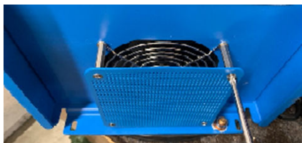
Figure 4 - 3kVA Blue Fan Cover Plate Installed
